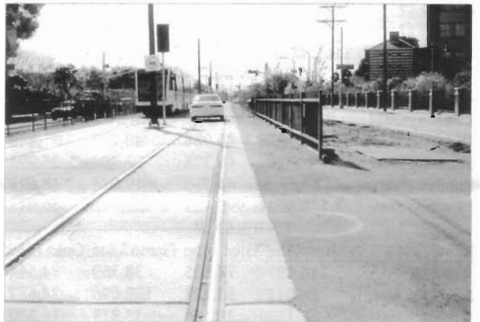
Light-rail vehicle on the Expo Line right-of-way on April 8, 2011, looking west. This was the first day of testing the LRVs under power. Previously, clearance tests were done by pulling the LRVs by giant high-railer trucks. Photo by Russ Davies
