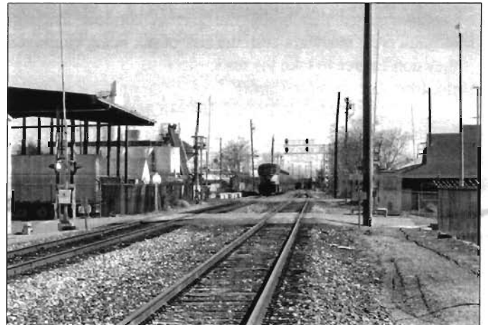
San Joaquin Train 714 is southbound on the BNSF Railway Stockton Subdivision after departing Stockton. The signals the train is approaching protect the Union Pacific Railroad Fresno Subdivision Crossing. Photo by Charles Varnes
