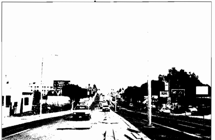
View to the east along 3rd St. is seen near McDonnell Ave., where Overhead Contact System poles are being installed within the new guideway. Metro and the Contractor are determining if vehicular access to properties can be improved as construction of the track guideway progresses. Image by Metro
