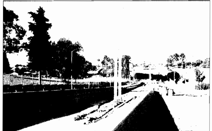
Gold Line Eastside Extension is seen to the west along 3rd St. near Sunol Ave., where the U-Channel section has been completed and Overhead Contact System poles are being installed within the guideway. Image by Metro
