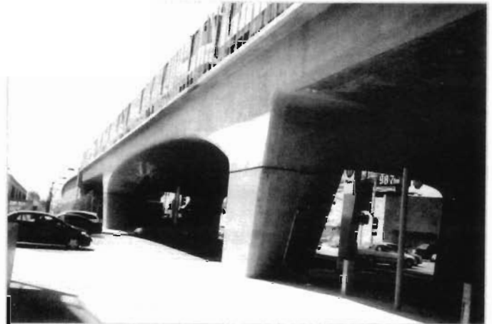
Expo/La Cienega Station with La Cienega Boulevard passing under center of station.
