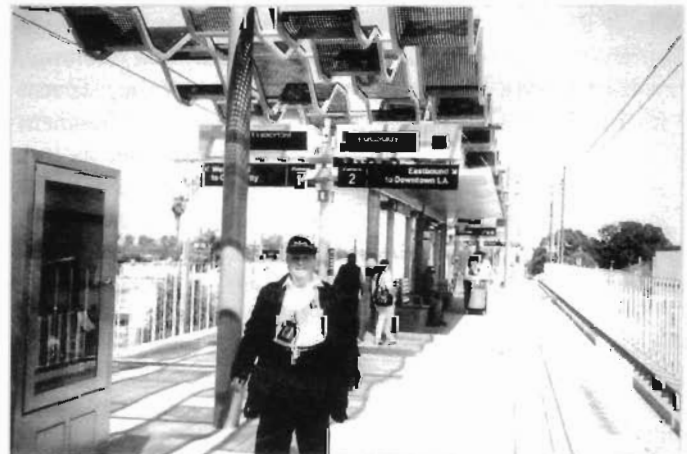
Expo/La Brea Station showing typical wavy sun screens with purple color above and aqua structure beneath.
