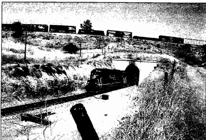
A Southern Pacific freight train passes underneath itself while descending the Tehachapi Loop grade in July 1965.
