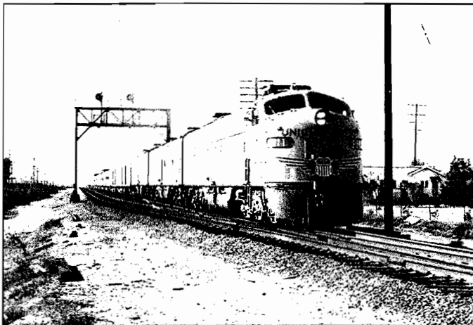
In her last year of operation in the spring of 1970, Union Pacific Train No. 104, the City of Los Angeles, is caught blasting eastbound in throttle position "run 8" after making a scheduled stop at the East Los Angeles Station. When Amtrak was inaugurated approximately one year later on May 1, 1971, Train No. 104 said adios and sadly exhilarated us no more. UP locomotive 911 then became Amtrak 416. Photo by John Petros
