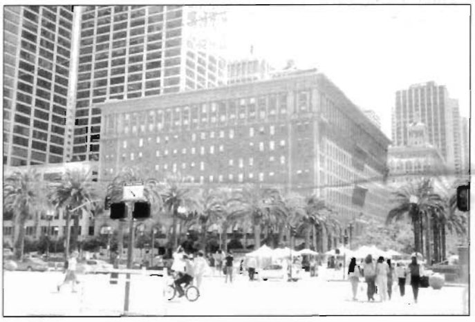
Old Southern Pacific headquarters building in San Francisco on August 9, 2006. Photo by Dennis Gilkey
