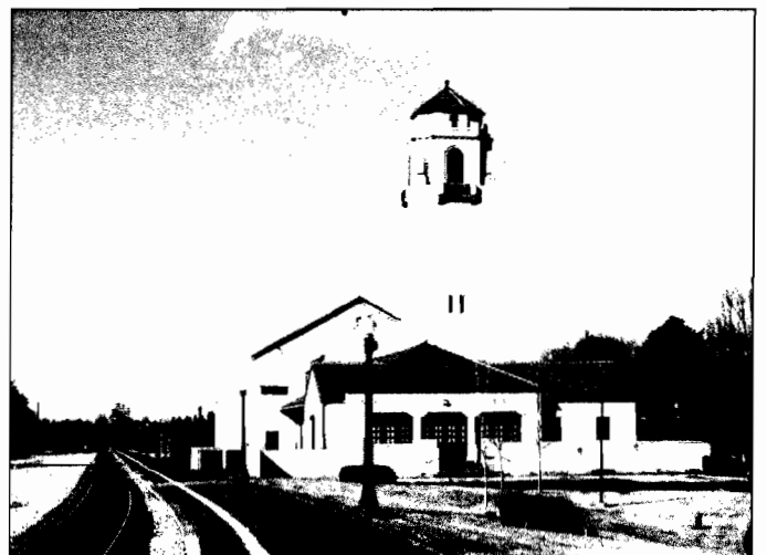
The beautifully restored Boise, Idaho, depot is seen in this picture on February 19, 2007. No longer used as a railroad depot, today the structure houses a museum and is available as a site for special events.
