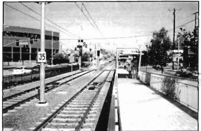
Expo/Crenshaw Station with westbound platform to east of Crenshaw Blvd. in the distance.
