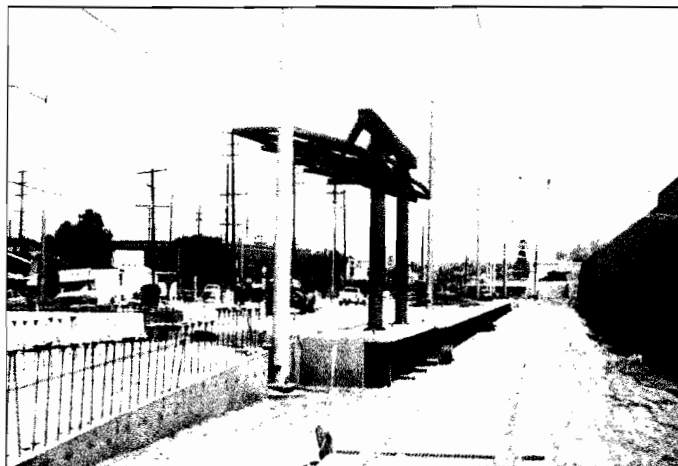
Installation of canopy on the Indiana Light Rail Transit Station platform on the east side of 3rd Street. Photo by Metro
