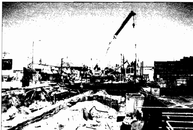
Concrete deck panels and steel deck beam removal over the 1st/Soto underground station. Photo by Metro
