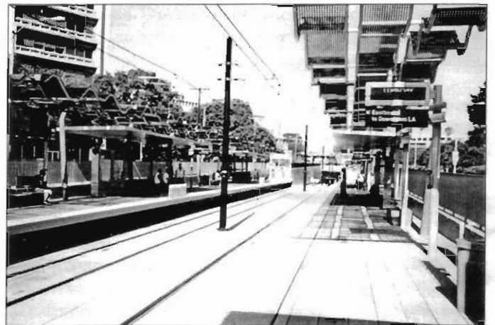
Expo Park/USC Station with eastbound platform to right of tracks and tracks leading toward tunnel beneath Figueroa Street. Photo by Dick Finley
