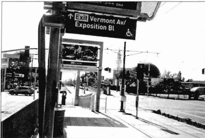
Exposition/Vermont Station with westbound platform beyond Vermont Ave. crossing. Tracks are in concrete. Photo by Dick Finley
