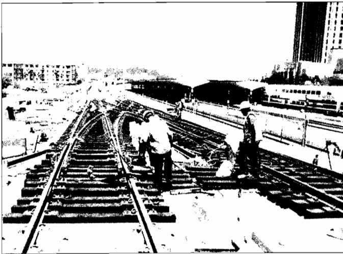
The tie-in of the Gold Line Eastside Extension to the Pasadena Gold Line is nearing completion. Photo by Metro
