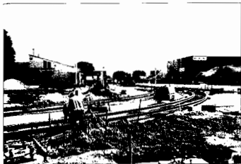
The Indiana Station and site work along the east side of Indiana progresses with track installation at the northeast corner of 3rd Street and Indiana Street. Photo by Metro
