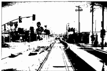
View from 1st Street LRT Guideway to West Portal is seen with construction of the track guideway and the Pico/Aliso Station under way. Photo by Metro
