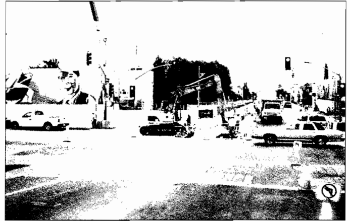
Construction of the 1st/Soto station underground structure and side structure surface penetrations are well underway. Relocation of utilities is being performed prior to the removal of the temporary concrete deck panels and street restoration improvements, scheduled to begin June 6, 2008. Photo by Metro
