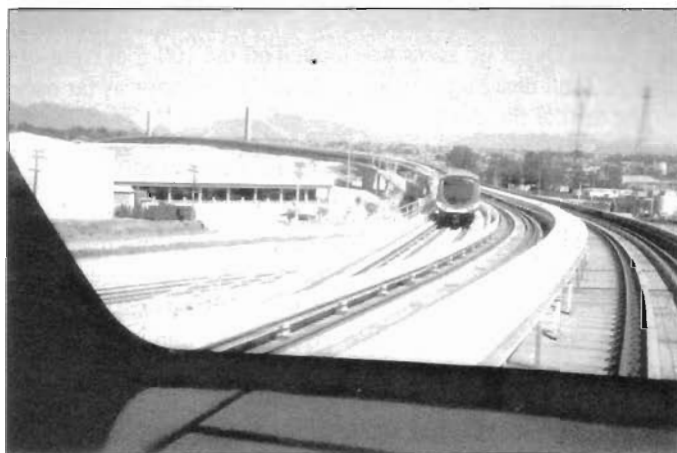
Northerly view in Richmond, British Columbia, where the "Canada Line" splits with one route to Brighouse station to the south, and the other showing the Vancouver Airport train dropping down to ground level to the west to pass under the flight approach. Trains cross the Fraser River on a cable-stayed bridge in background. Photo by John L. Whitmeyer
