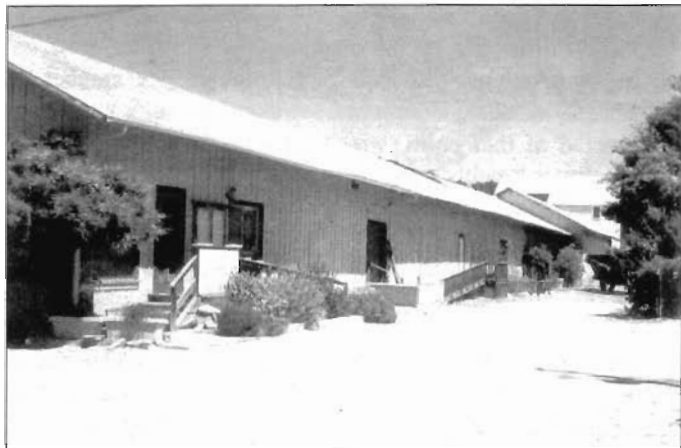
The former Pacific Coast Railway station in Los Alamos, CA shows the west facing facade and south along the removed road-bed. This was mainly the freight house of the three-foot narrow gauge operation which was abandoned in December 1941. The PCR ran from San Luis Obispo to Los Olivos, CA crossing the Southern Pacific at Hadley (south of Edna). It had branches to Port San Luis and to Guadalupe. Photo by John Petros
