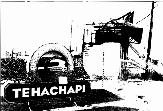
The south end of the 104-year-old Southern Pacific depot is all that remains following a June 3, 2008, early morning arson-caused fire. Photo by John Ulloth
