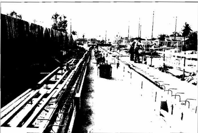
Indiana Station construction near 3rd St. is well underway. Photo by Metro
