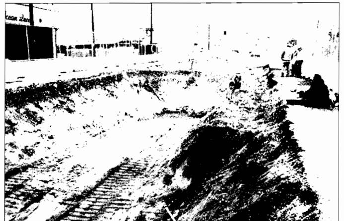
Excavation for construction of the Pico/Aliso Station near 1st/Utah has been completed.
