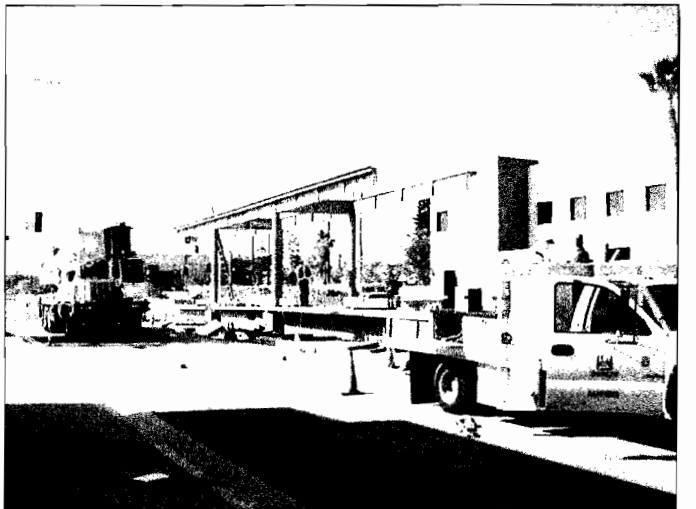
The Overhead Contact System and station canopy are being installed at the Atlantic Station at Pomona/Atlantic Blvds. Photo by Metro
